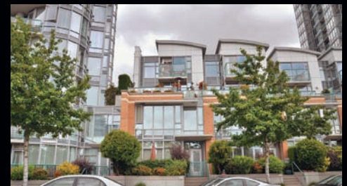
QUAYWEST RESORT 3F - 1067 Marinaside $1,999,000
