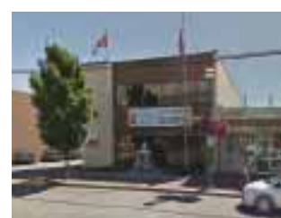
5,286-square-foot office building, previously a Royal Canadian Legion, Langley, sold for $1.52 million. | NAI COMMERCIAL
