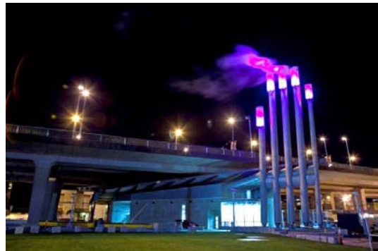
Southeast False Creek Neighbourhood Energy Utility.
