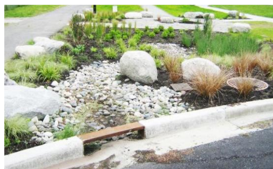
Rain gardens are planted areas behind curbs that filter stormwater from the street.
