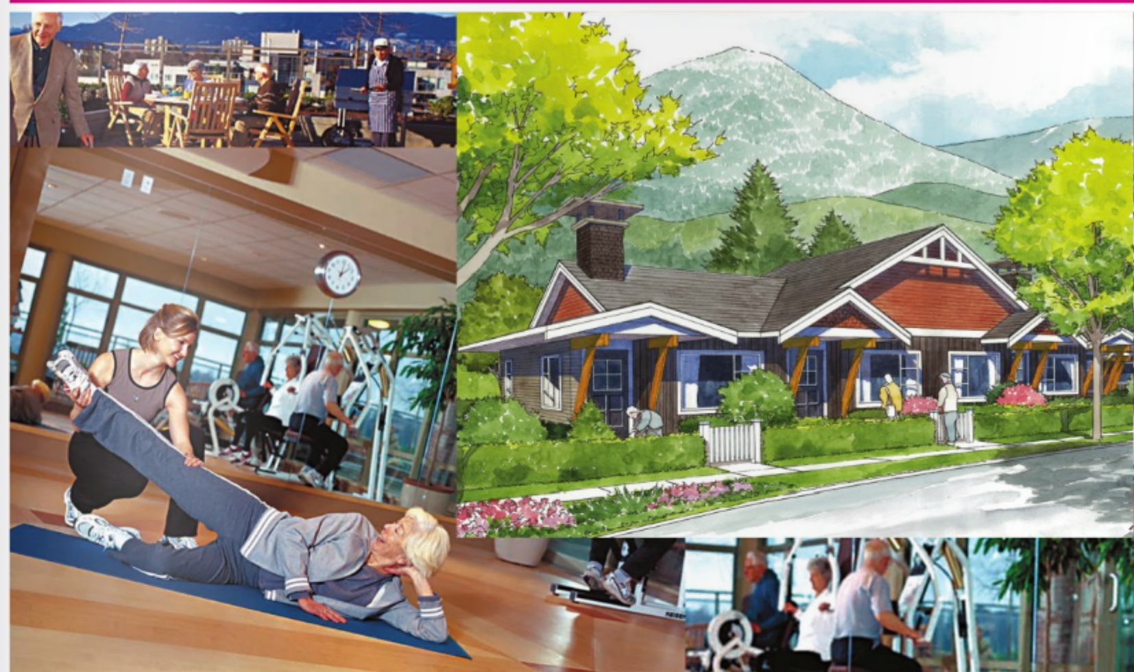
SENIORS FUTURE: Pre-fabricated, one-level strata units, such as these proposed by the Keremeos Modular Housing for Seniors project, are potential examples of the future of B.C. housing as older buyers dominate sales. Photo: Scuka/BC Housing
