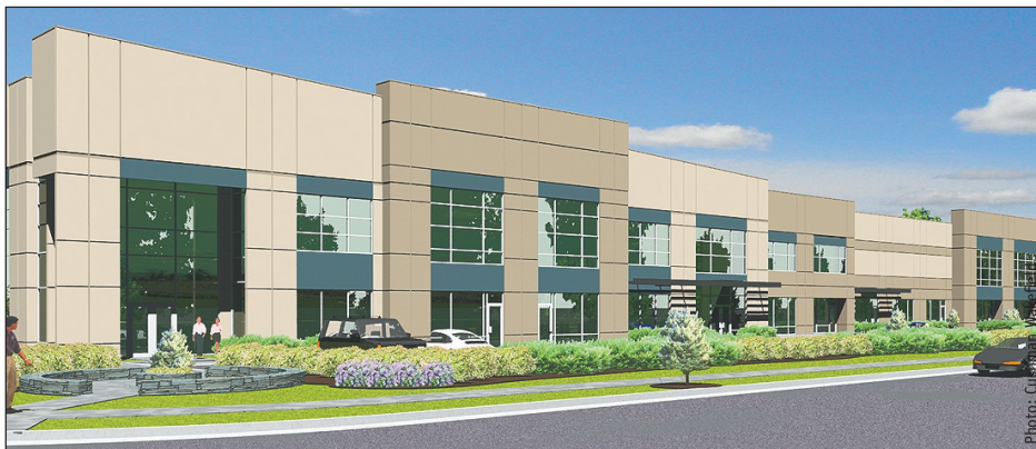
Industrial strata space now accounts for 38 per cent of the Metro Vancouver market and one-third of sales in Edmonton. Some spec builders aim to sell, not lease, in Calgary.
