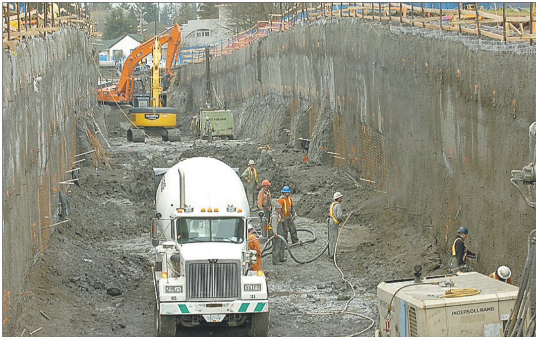
A truck carrying concrete (left) backs into the second section of a cut-and-cover tunnel that will run up Cambie Street. The tunnel is being lined with reinforced concrete to stabilize the walls. Workers (below) lay the concrete reinforcing bar that will form the bed of the new cut-and-cover tunnel under Cambie Street.
