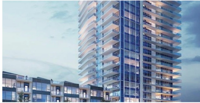
ASSIGNMENT AT IMPERIAL METROTOWN 402-5051 IMPERIAL STREET $799,000
