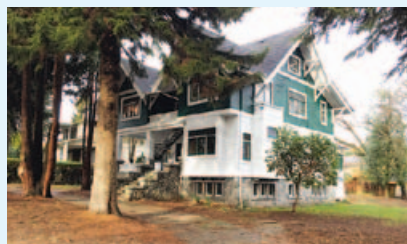
1033 Balfour Ave., Shaughnessy, Van $6,380,000
